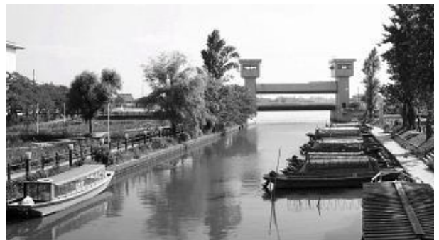
Figure 4. Changed into straight concrete lines.
